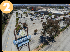
2 NORTHDRIDGE MALL (PARKING LOT)
