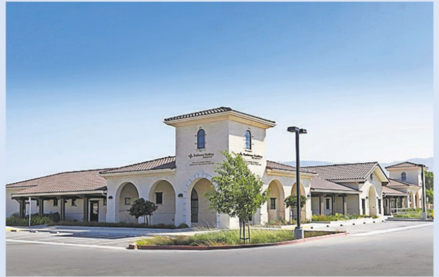
Salinas Valley Health's Taylor Farms Family Health & Wellness Center's 20,000-square-foot facility at 850 5th St., in Gonzales.
