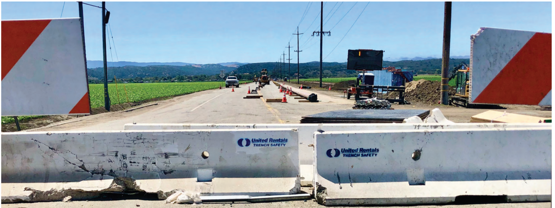
A natural gas pipeline on Davis Road in mid-August.
