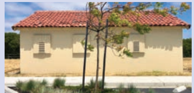
Fort Ord officers’ mess halls and latrines, built in the 1940s by the Works Progress Administration (WPA), will be renovated for reuse as artist studios for the Arts-Historic District in the East Garrison neighborhood at the former Fort Ord.
