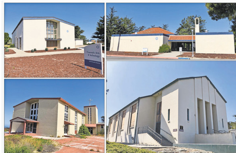
All four Cold War chapels still remain on Fort Ord as of the summer of 2025, although one is scheduled for demolition and another has been boarded up for years. Clockwise from top-left: Sixth Avenue Chapel, Bayview Chapel, Post Chapel, Durham Road Chapel.
